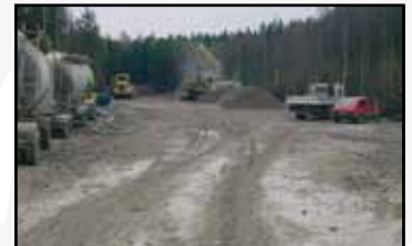
The swamp one week after stabilisation
